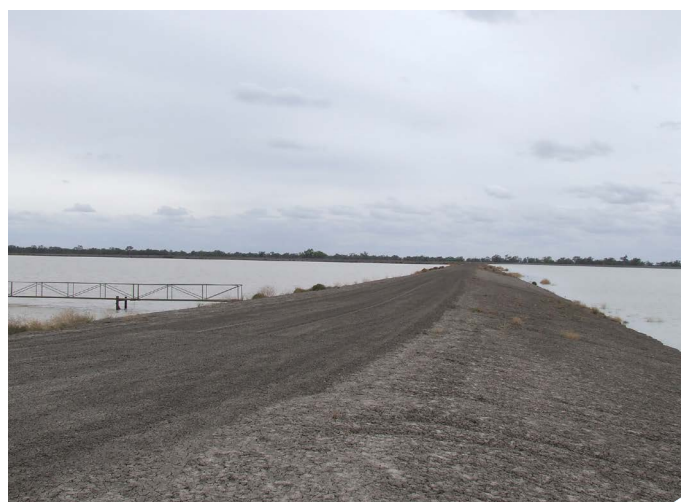
An on farm water storage split into cells to reduce evaporation (Image: J. Montgomery)
