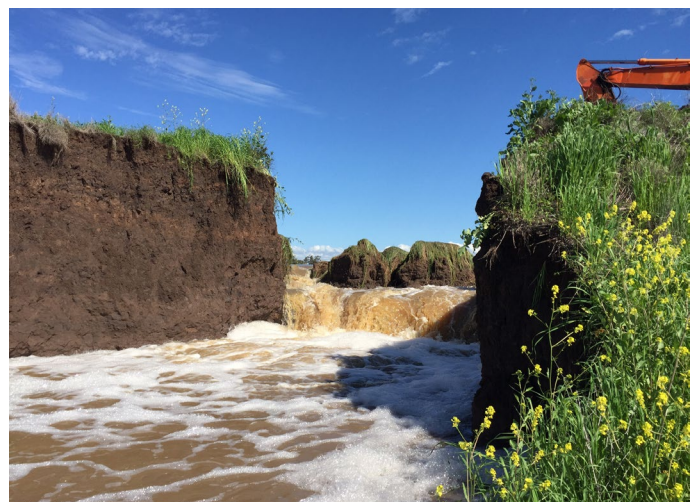
Failed storage (photo: STBIFM)
